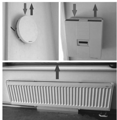
Fig. 3. Tested pair-wise, monoblock and ventilation radiator units in nearly zero energy test building.
