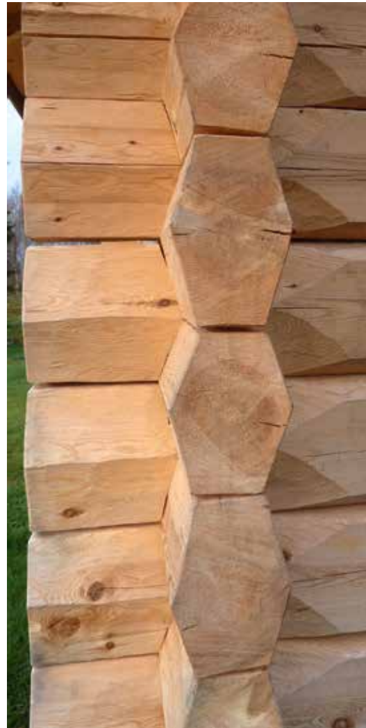
A log wall with the hex notch ( sulkanurkka in Finnish). Photo by Janne Jokelainen.
