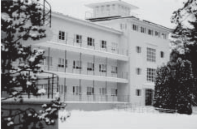
Modern renovated tuberculosis hospital: Kose Department of SA North Estonian Regional Hospital
