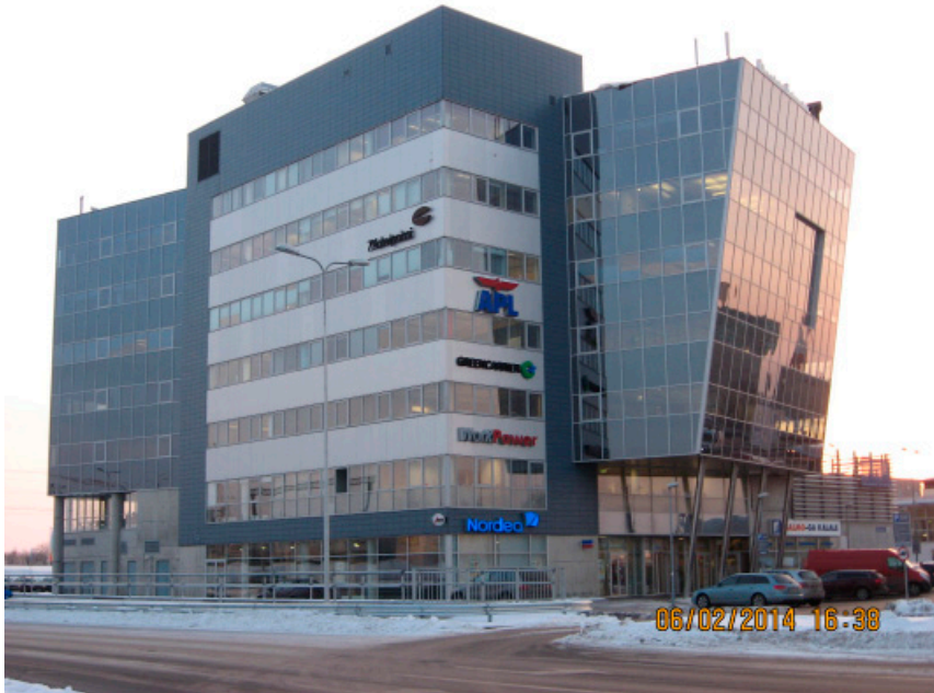
Joonis 1. Rippuva fassaadiga hoone Peterburi teel Tallinnas Figure 1. A self-shaded façade in Tallinn at St. Petersburg Highway
