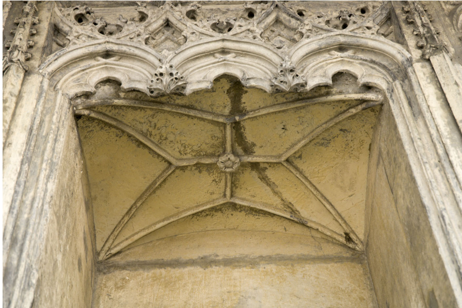
Fig. 7. Ceiling of the central niche with the imitation of the stellar vaults of the church. Photo by Stanislav Stepashko.
