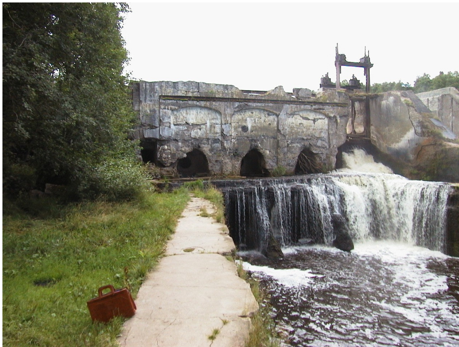
Figure 2. Linnamäe, a year before the rehabilitation
