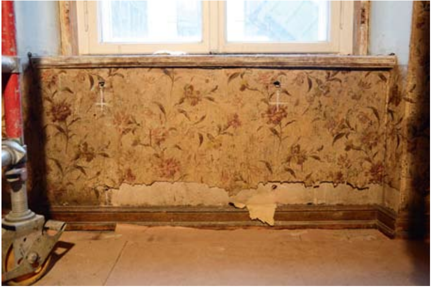
Figure 157. Area of wallpaper from behind the radiator before its removal.
