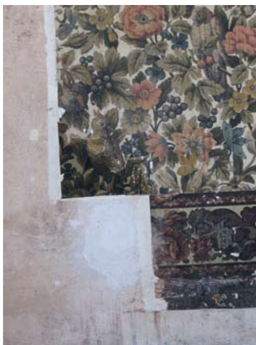
Figure 180. Small missing areas were filled with the wallpaper fragments found behind the wooden overdoors.
