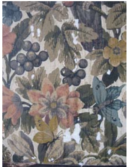
Figure 94. The minor losses in the surface of the wallpaper found in the dining-room of the Puurmani manor were filled with a fine layer of applicable paper paste.
