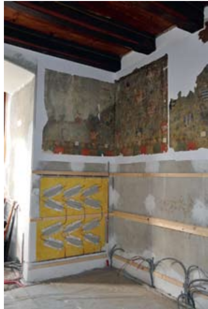
Figure 128. Wallpaper fragments during and after remounting.
