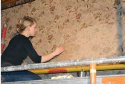
Figure 159. Two main colours of the pattern were printed with stencils.
