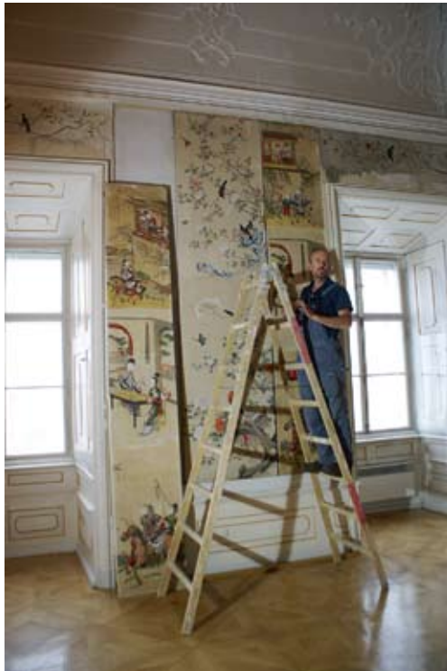
Figure 143. All the panels carrying the wallpapers were dismantled from the wall.
