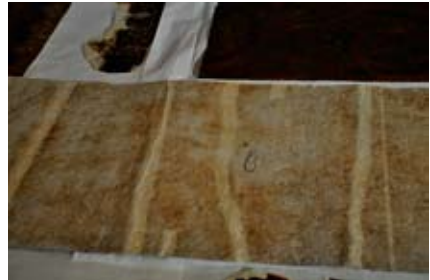
Figure 82. Removing heavy wallpaper from up downwards could result in numerous cracks and damaging the layer of paint.
