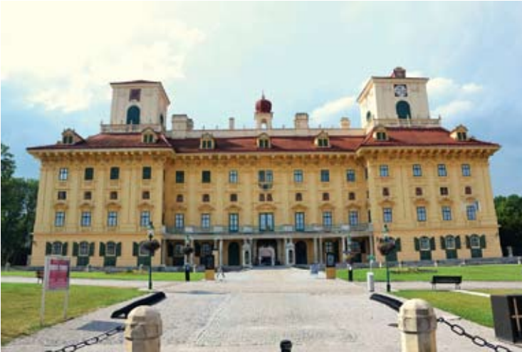
Figure 141. Esterházy Palace in Eisenstadt, Austria.
