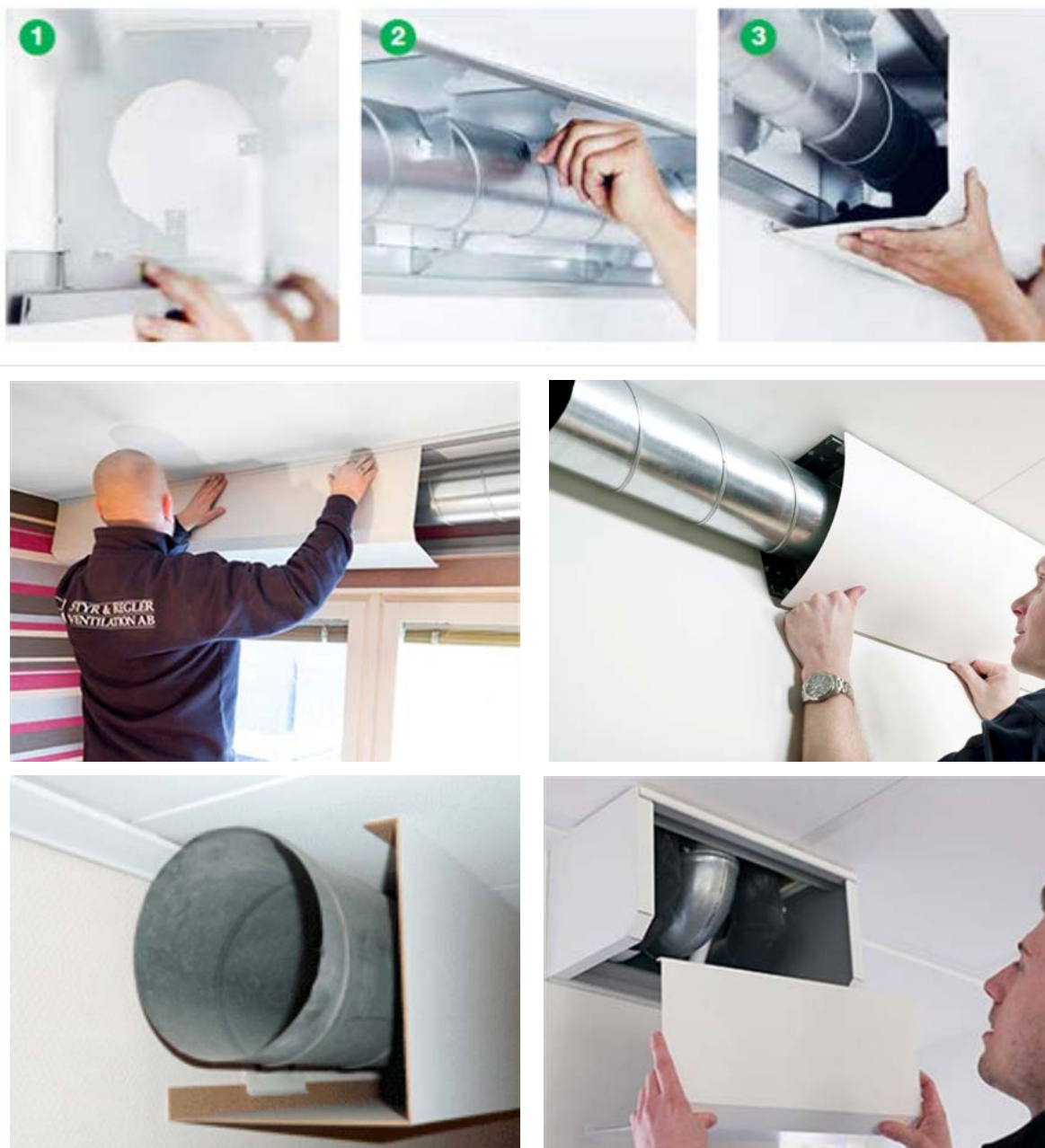
Joonis 3.19 Ventilatsioonitoru korteris paigaldatakse spetsiaalkarbikusse (Lindab InCapsa: www.lindab.com , \\liab.lindab.com\LinFiles\Company\79AII\Incapsa\Lindab_Master_110714_2_h264 Montering.mov, https://www.youtube.com/watch?v=C2AREepzlrk ; https://www.youtube.com/watch?v=gVI0Rc15QU4 , Hallstroms INTERIOR: http://www.hallstroms.com/wp/produkter/hitac-interior/?lang=en ).
