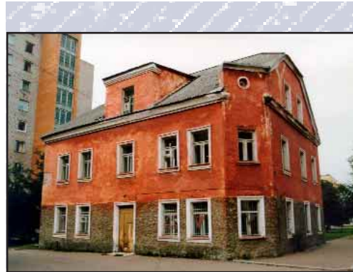
The house in Narva before repair works ...
