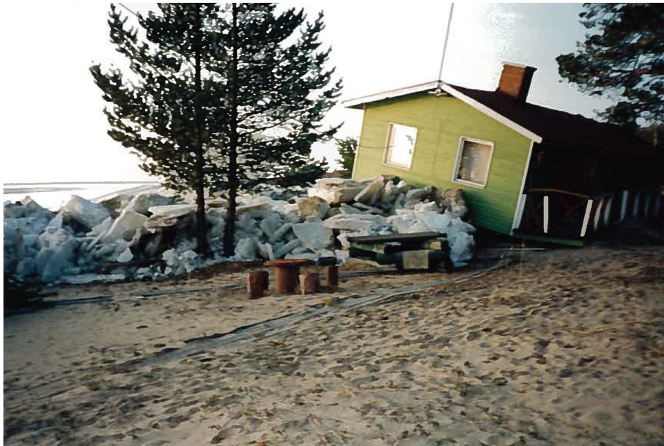
Fig. 6. Ice ride-up on the shore in Hailuoto on 19 December 1992: A , ice sheet breaks onshore; B , ice pushes a house close to the shoreline. © Courtesy of Mr Markku Tönkyrä, Hailuoto.
