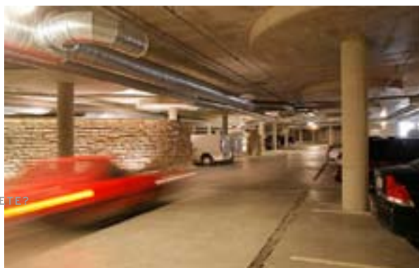
Underground car park
