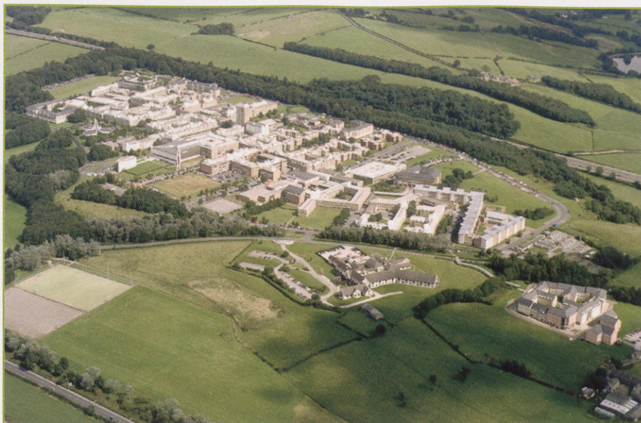
Anneli's future campus in Lancaster.
