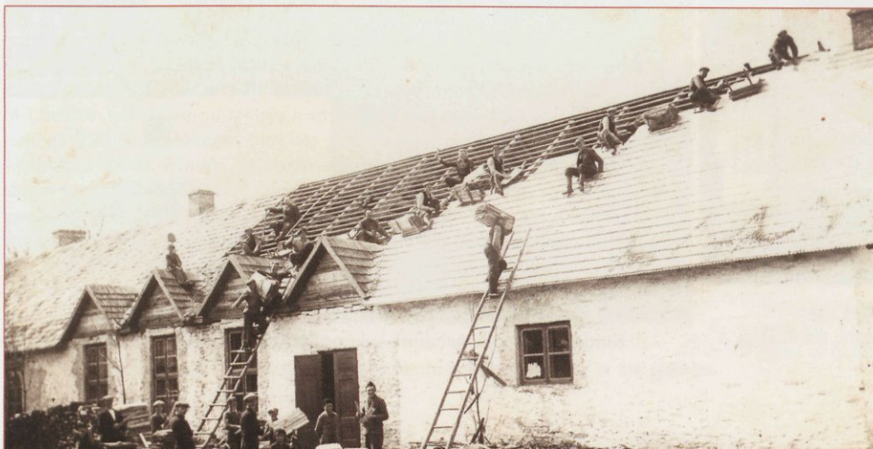
Rahvamajale uue laastuka- tuse lõõmine Raplamaal Kabalas, umbes 1930. The local community centre is getting a new shingles roof. Kabala in Rapla County, about 1930.
